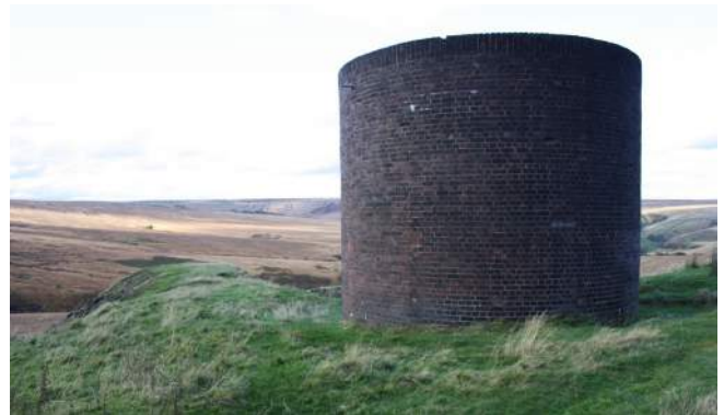
Figure 2: A canal ventilation shaft at the head of the Upper Colne Valley. Canals built over, under and into the Pennines opened up the landscape in the 19th century, allowing transport of raw materials in and out of the valleys © Minerva Heritage Ltd.
