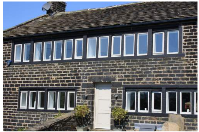
Figure 1: The Castleshaw and Upper Colne Valleys still contain dozens of examples of woollen workshops, some now converted into residential dwellings but many more of which have been lost. The small windows lit up the looms of the 18th-19th century weavers © Minerva Heritage Ltd.
