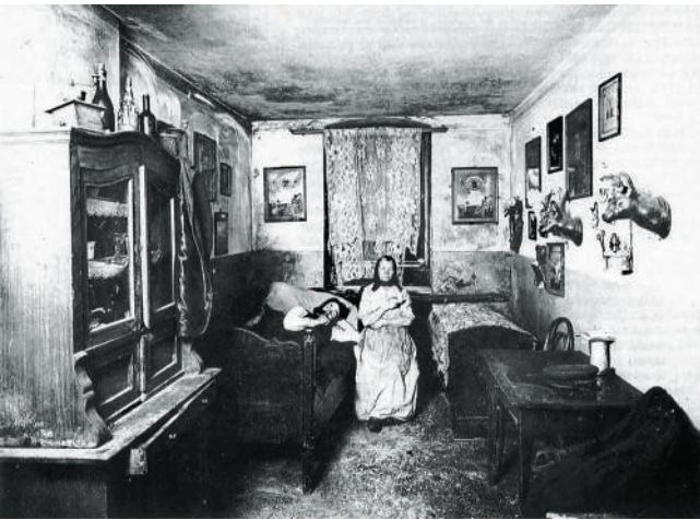
Figure 2: A basement apartment in Berlin from 1908. The description of the apartment states: "Through the old door in bad condition one gets into a poorly furnished apartment. The whitewashed walls of this room are completely covered with smoke. The room height is 2.60, out of which 1.95 are below street level. The window is 1.15m." Source: Geist, J.F./ Kürvers, K. 1984. Das Berliner Mietshaus 1862-1945 . München, p. 462.)
